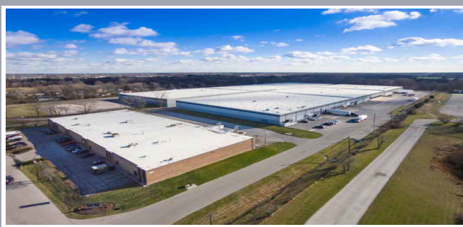
Franklin Road Distribution Center , Indianapolis, IN, $15,200,000
