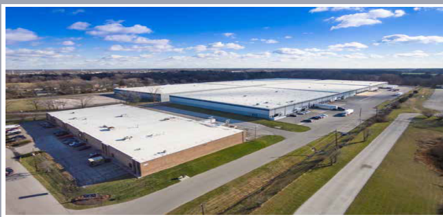
Franklin Road Distribution Center , Indianapolis, IN, $15,200,000
