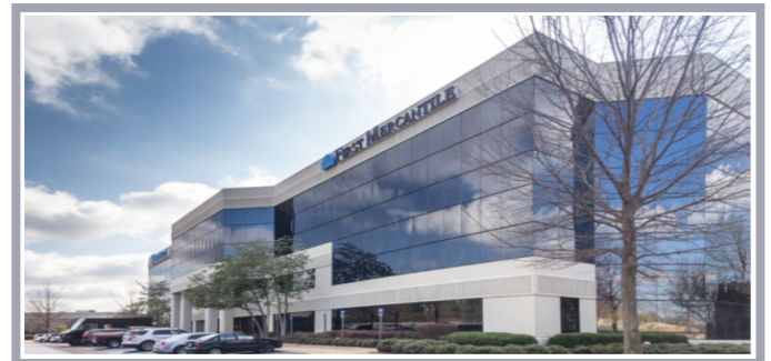
Germantown Park Offices , Memphis, TN, $47,750,000
