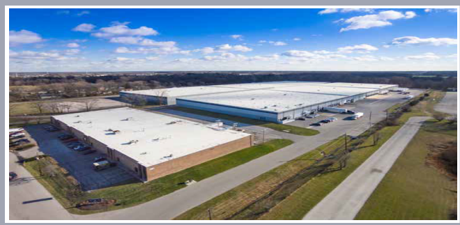
Franklin Road Distribution Center, Indianapolis, IN, $15,200,000
