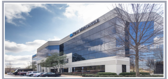
Germantown Park Offices, Memphis, TN, $47,750,000
